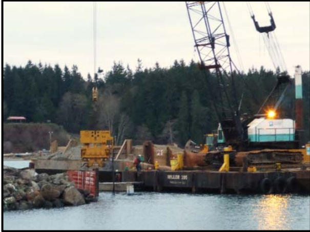
Demolition of the transload facility.
