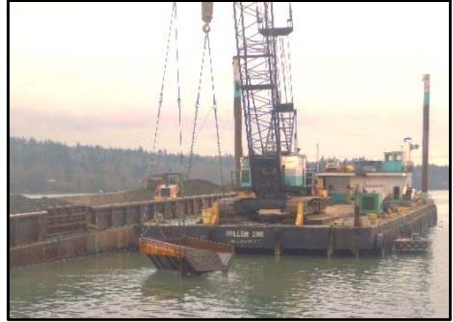
3" minus backfill being placed with a 10 cubic yard capacity rock box.
