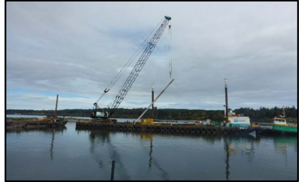
Installation of temporary piles for the SMA-1 loading/mooring facility.
