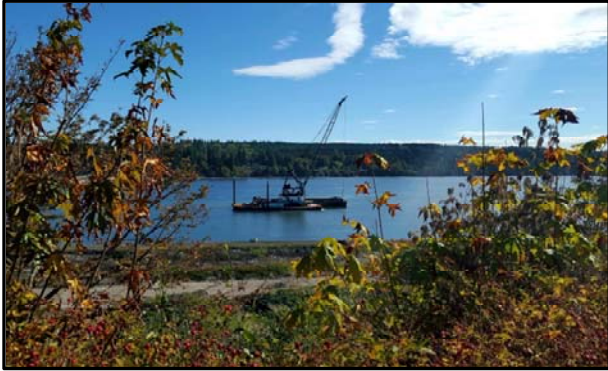
Large crane and barge set up ready for dredging.
