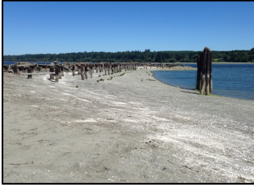
Before Cleanup: SMA-1 intertidal area, jetty towards the north end of the millsite.
