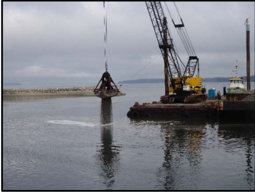
Clean capping material being placed in SMA-1.
