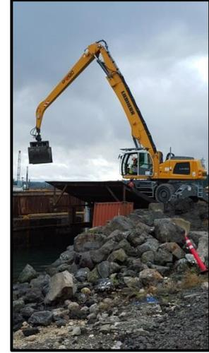
*Subtidal dredge spoils being offloaded from a barge.*
